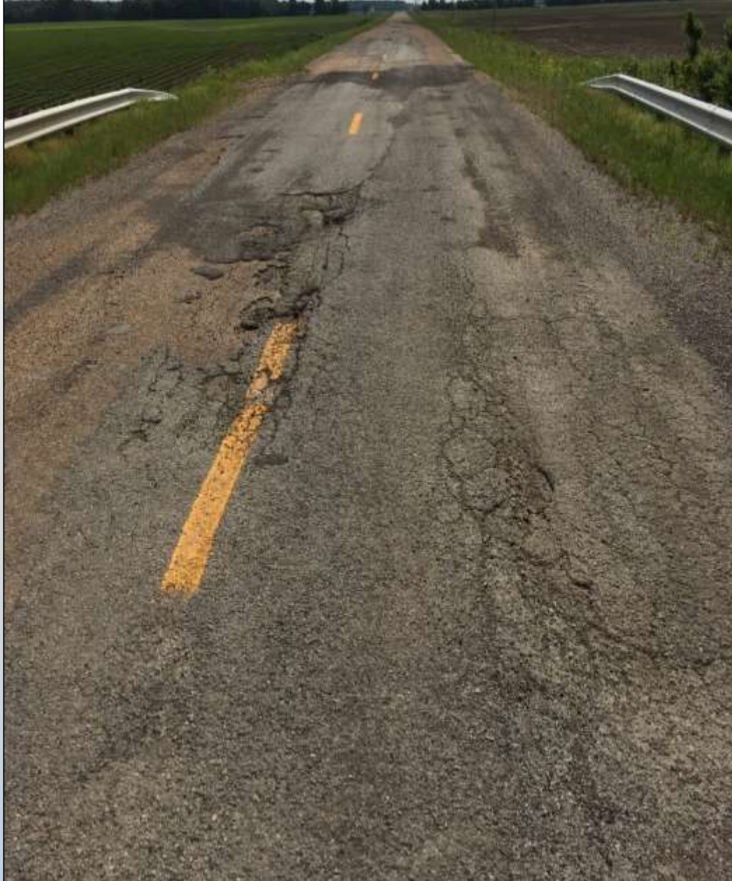
Mississippi County Highway 34 East of Highway 77
