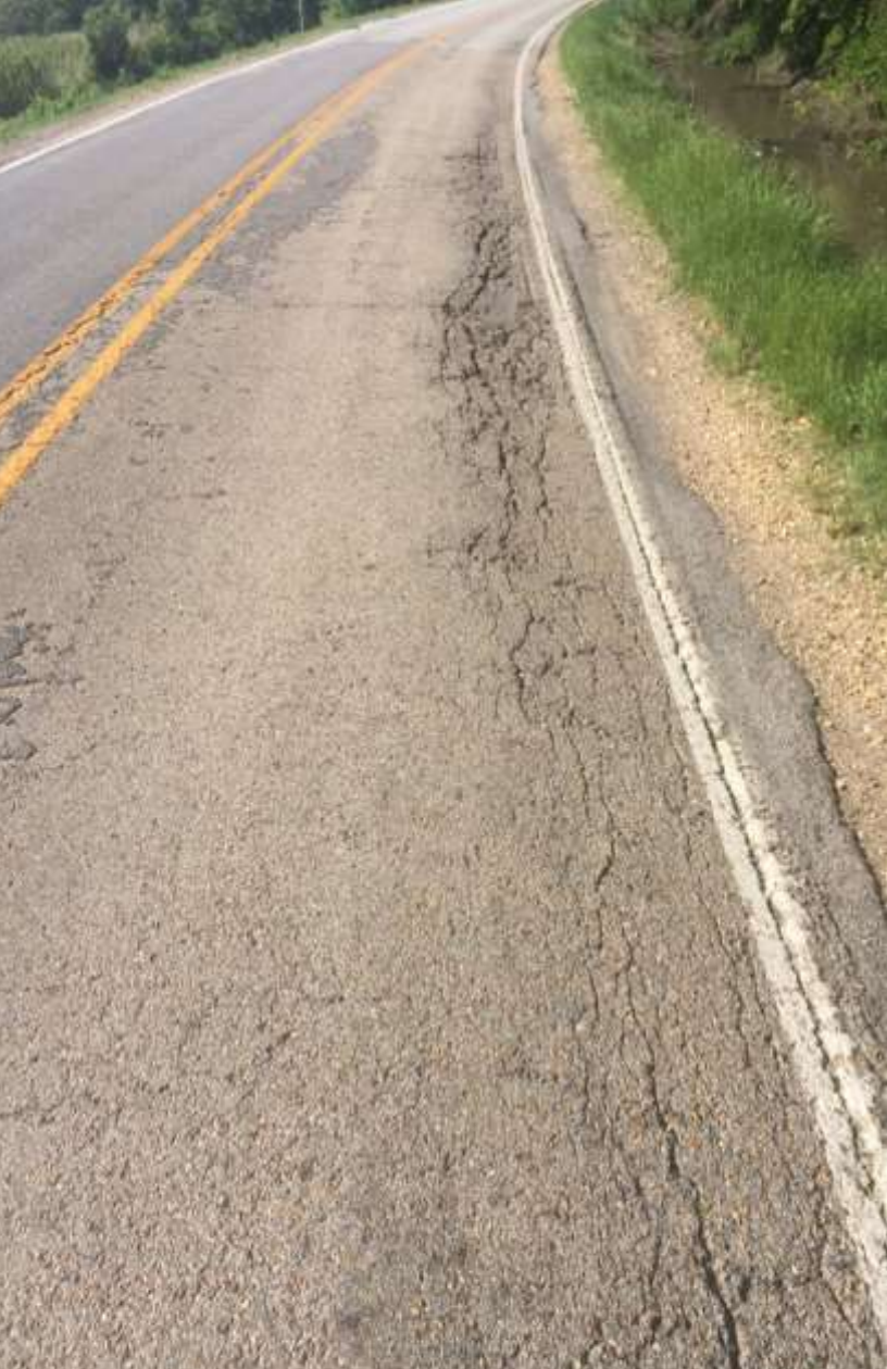
Lawrence County Highway 34 Near Okean
